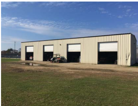
Figure 8(a) – Existing Facilities Building
