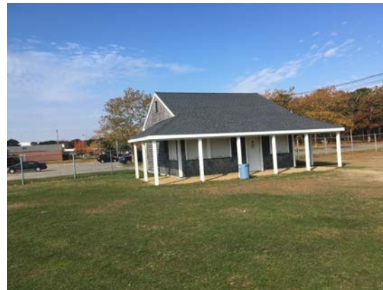
Figure 8(b) – Ticket & Concessions Building
